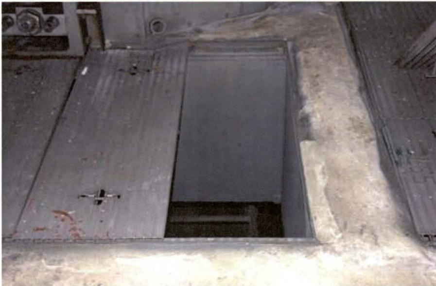
**Figure 43. LC 17B Exhaust Port on Launch Deck**
