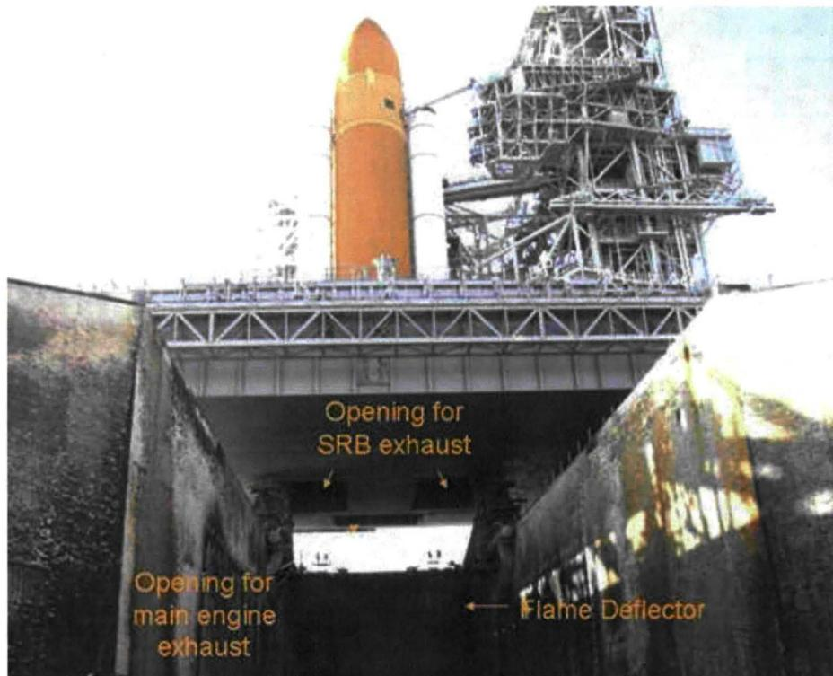
**Figure 4. Openings for Flames From the Main Engine and SRBs**
