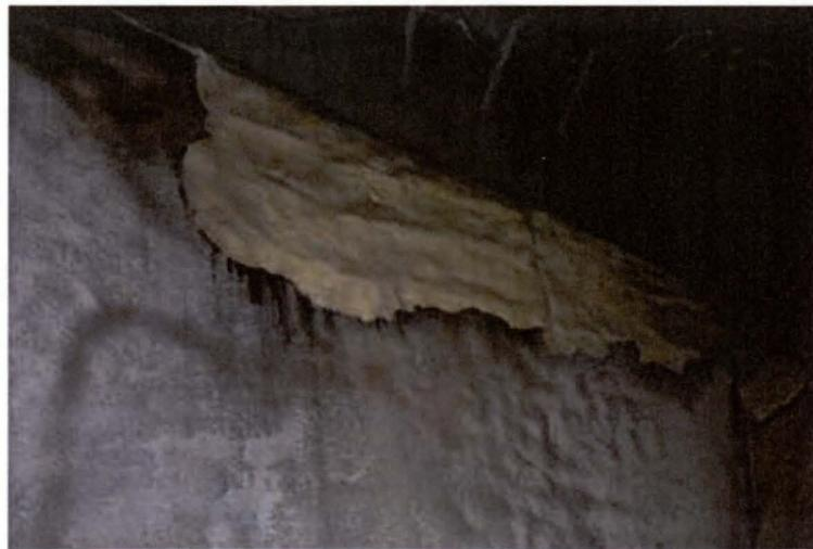
**Figure 39. Martyte Patch on Flame Deflector Side Wall**
