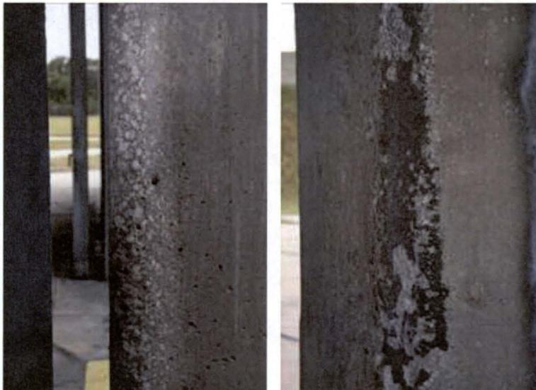
**Figure 35. Damage to Side Flame Tunnel Support Columns**
